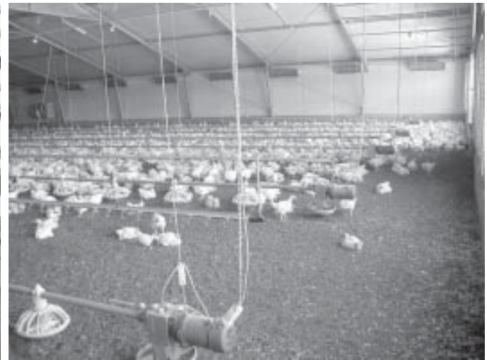
This 80-foot wide tunnel ventilated house in Australia has five feed lines. Note the number, size and location of the sidewall inlets for cool weather ventilation.
