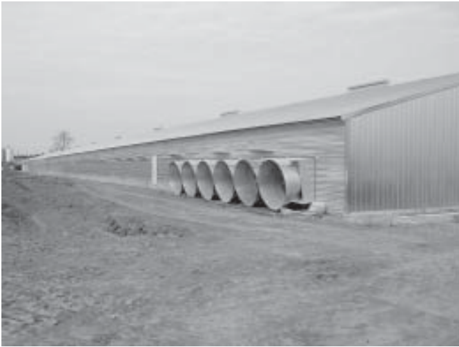
When buildings get wider, the number of tunnel fans and the amount of evaporative cooling pad must increase to handle the volume of air necessary for good ventilation. This clear-span 66 x 500 ft building utilizes all-steel construction technology for trusses and walls.
