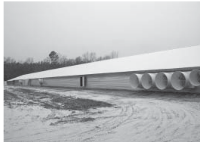
This 60 x 500 foot wood truss building under construction will be ready for birds within the next few weeks. Because good airflow is essential, note that all fans, both tunnel and sidewall, are slantwall cone fans with high airflow ratings.
