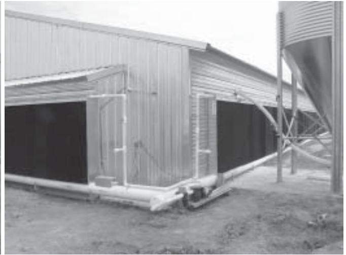
When buildings get wider, the number of tunnel fans and the amount of evaporative cooling pad must increase to handle the volume of air necessary for good ventilation. This clear-span 66 x 500 ft building utilizes all-steel construction technology for trusses and walls.
