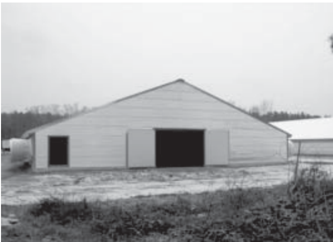
This 60 x 500 foot wood truss building under construction will be ready for birds within the next few weeks. Because good airflow is essential, note that all fans, both tunnel and sidewall, are slantwall cone fans with high airflow ratings.
