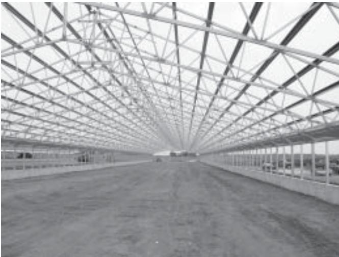
This wide building utilizes poured curb foundations and tubular steel structure.
