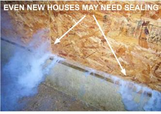
Cold air entering through cracks or doors, vents or shutters that don't shut properly hurts static pressure and spoils the airflow pattern needed for cold-weather ventilation. Smoke testing during a pressure test is a good way to find unsuspected air leaks. Air can enter a poultry house in places that you would never expect. Even new houses benefit from smoke tests; we frequently find leaks in newly built houses as well.
