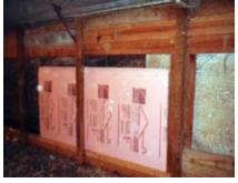
The picture on the left shows one way of sealing off an unused fan for the winter to cut down on heat loss and unwanted air entering. A second curtain can be installed on the interior side of the tunnel inlet for added protection from air leaks. Board insulation can also be added to most any tunnel inlet to help add some R-value to that area of the house.
