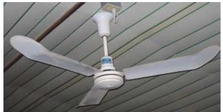
Stir fans reduce temperature stratification by thoroughly mixing in-house air during and between minimum ventilation run times. Almost any house will benefit from the addition and proper use of stir fans during wintertime. Almost any house can benefit from stir fans, but the benefits are more pronounced in older houses that are loose, have curtains and have high ceilings.
